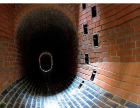
Figure 5 Connection to the “K” interceptor (1200/1800 mm profile)
