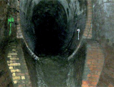
Figure 2 Original overflow chamber – “frog mouth”
