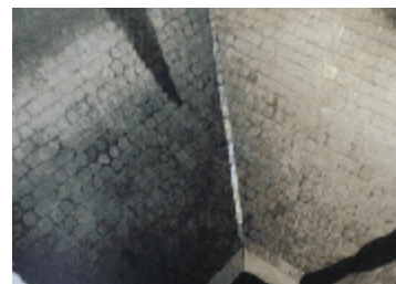
A Power Station Coal Bunker completely lined in cast basalt tiles
